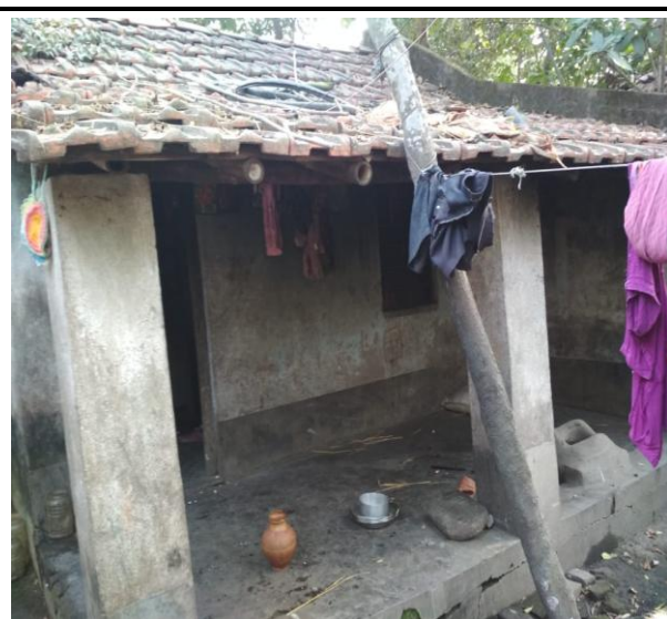
Picture 1: Shelter and latrine
