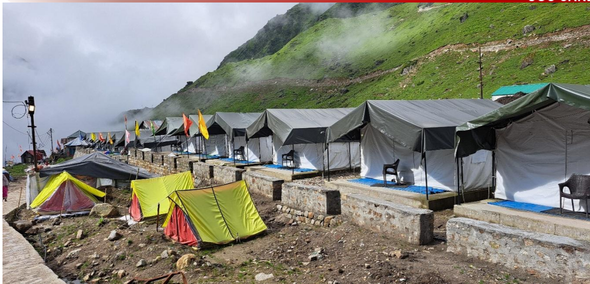
Photo 8. Garhwal Mandal Development Corporation's excavation of meadows and installation of permanent, cement-based tents. These tents have ruined the natural beauty of 'bugyals'
