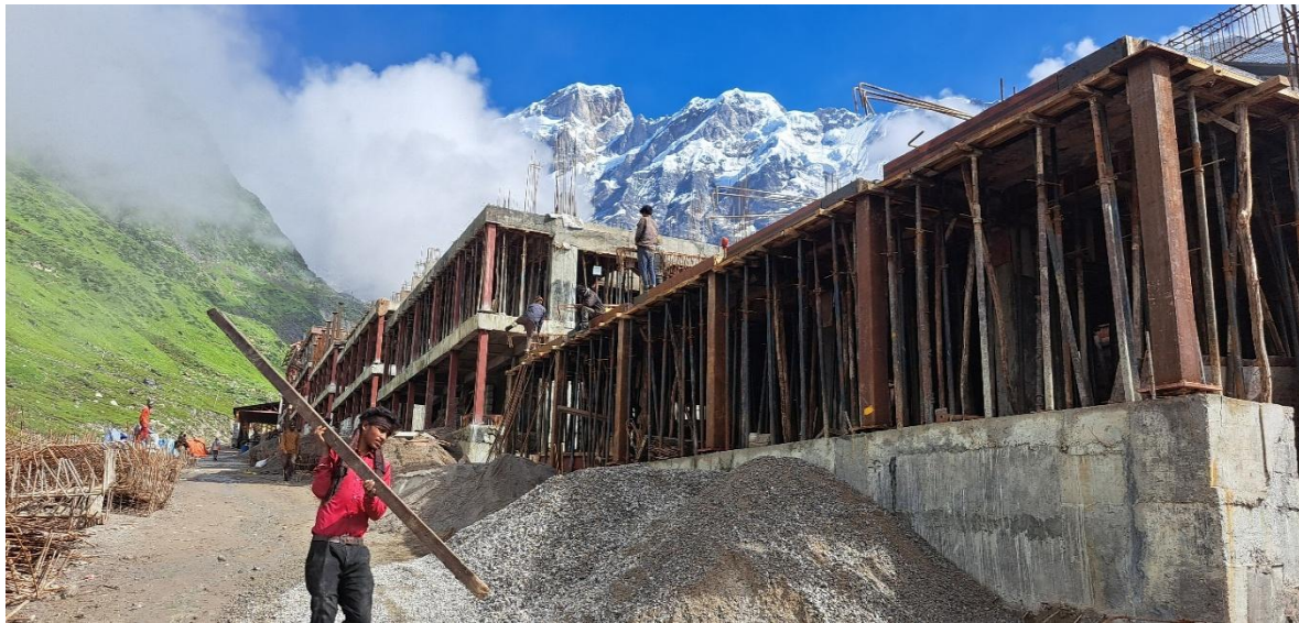
Figure 6. New structure coming up in Kedarnath town. Over-construction has led to the “concretization” of open spaces.
